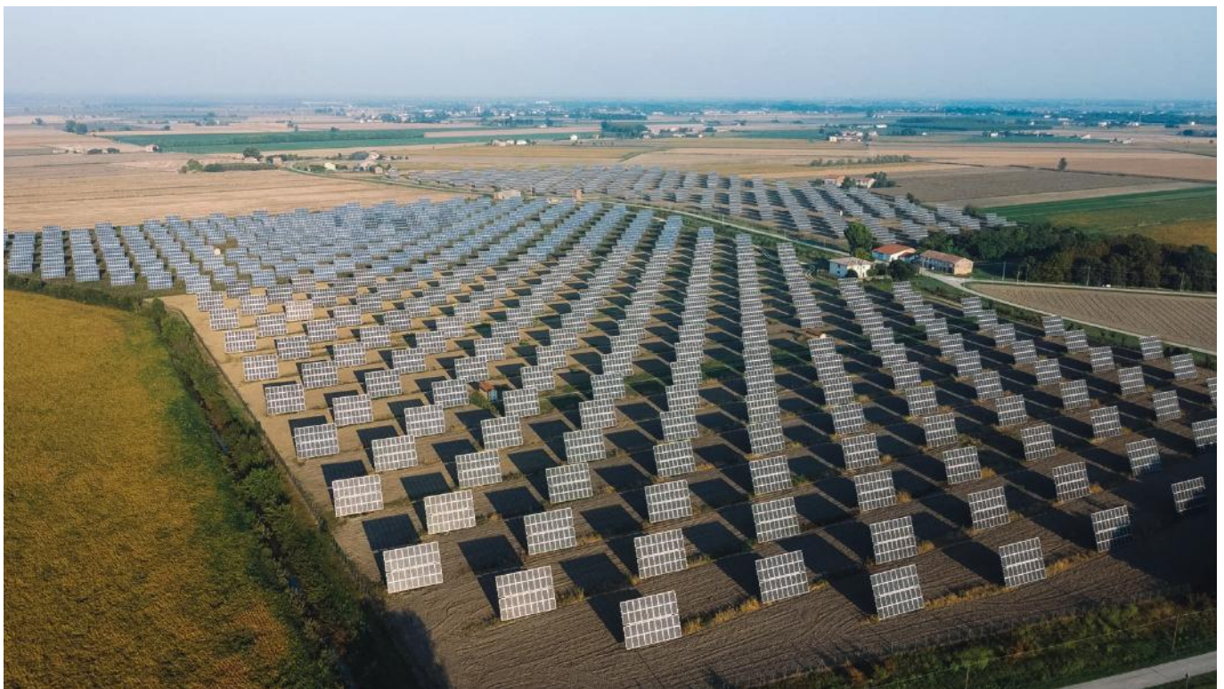
Photovoltaic system near Castelguglielmo (IT)
