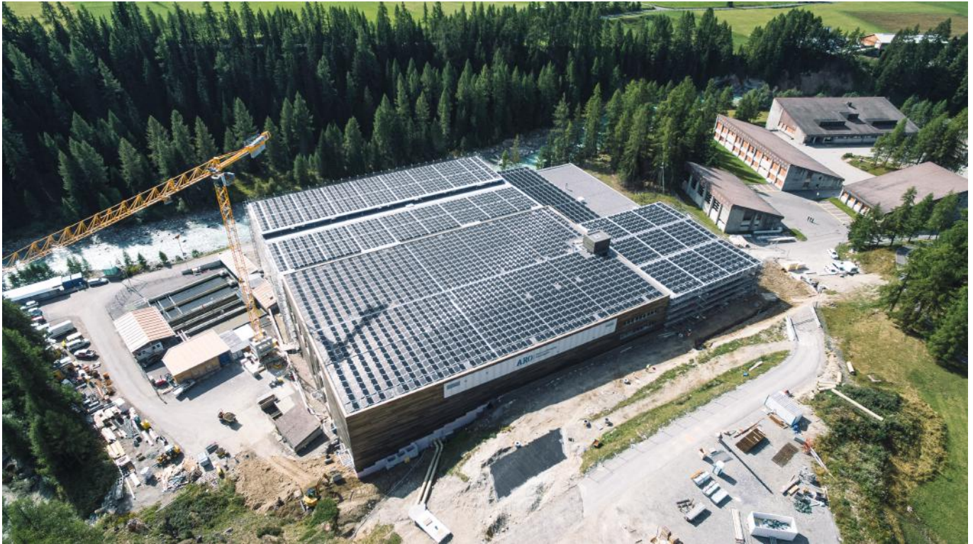
Photovoltaic installation on the roof of ARA Oberengadin sewage treatment plant
