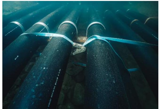
The cable conduit is first run along the surface of the lake before being lowered to the bed, supervised by professional divers.
